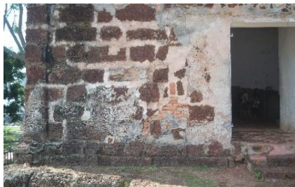
Figure 8: Usage of brick for stone replacement
