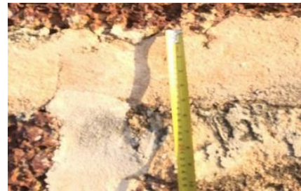
Figure 9: Pointing technique, 50-100mm of thickness
