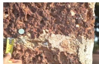
Figure 4: Early mortar for jointing material
