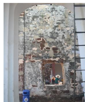
Figure 10: Mortar patch over the laterite surface
