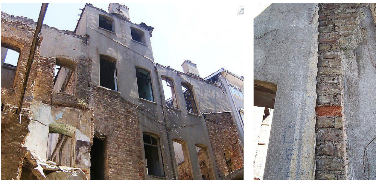
Figure 2. Traces of the wooden structures at the rear facade of the main building; photo by H.A. Doğan. (Doğan 2023)
